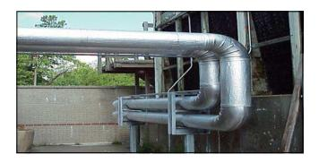
Alumaguard® All-Weather should only be applied to faced fiberglass or faced closed-cell foam insulation board.
