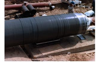
**INSULRAP™** 50 NG is the "Next Generation" premier direct burial membrane in the insulation market used as a waterproofing and vapor-proofing jacket. It is the first jacket of its type offering true zero perm performance.
