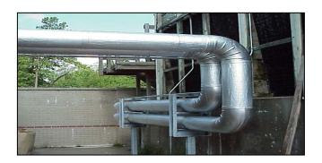
Alumaguard All-Weather is typically applied to faced fiberglass board, rigid isocyanurate foam board with facing, or unfaced extruded polystyrene foam board.
