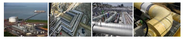
**Insulrap**<sup>™</sup> **JB** is a self-adhesive multi-layer white PET/FOIL/PET zero perm membrane designed specifically for LNG and Cryogenic insulation systems. The product is constructed of a proprietary Polyguard butyl compound, which is a peel and stick self-sealing with excellent low temperature adhesion and flexibility.
