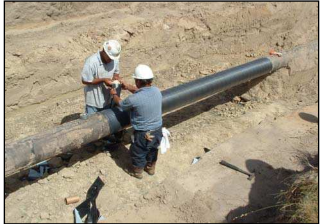
INSTALLING OUTERWRAP
