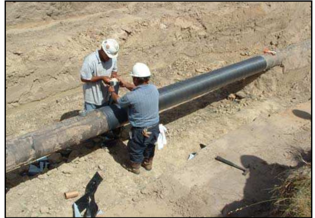
INSTALLING OUTERWRAP
